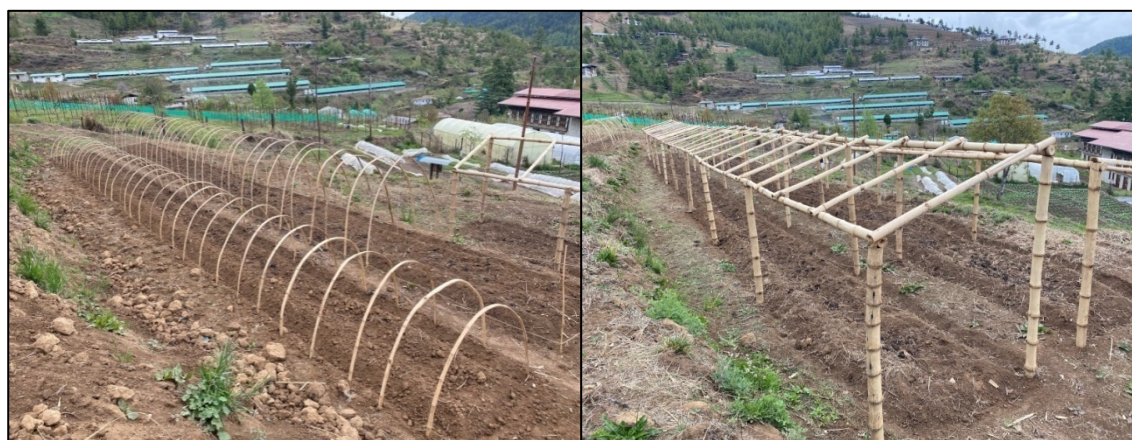
Figure 45: Two types of rain shelter frames constructed with bamboos
